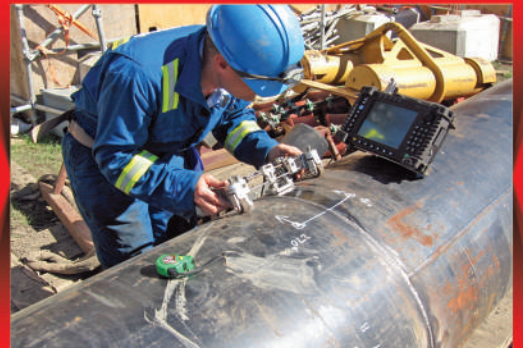
Automatic Ultrasonic Weld Inspection
